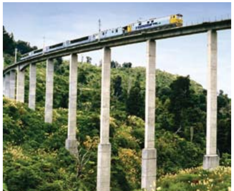
Overlander on viaduct
